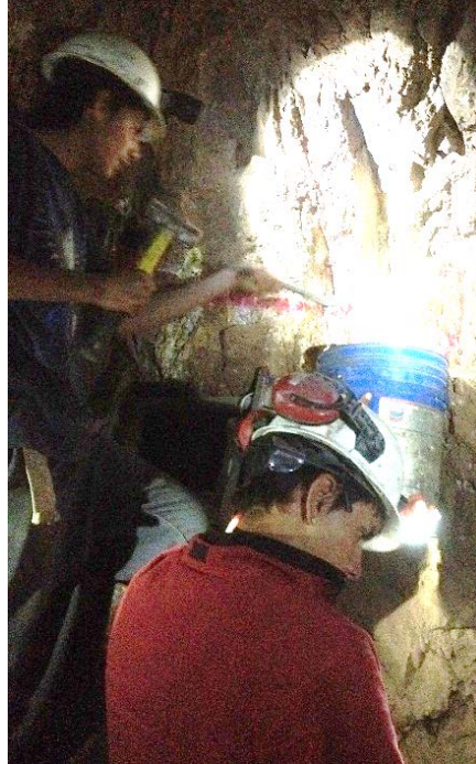
Figure 11-2: Channel Sample Collection
